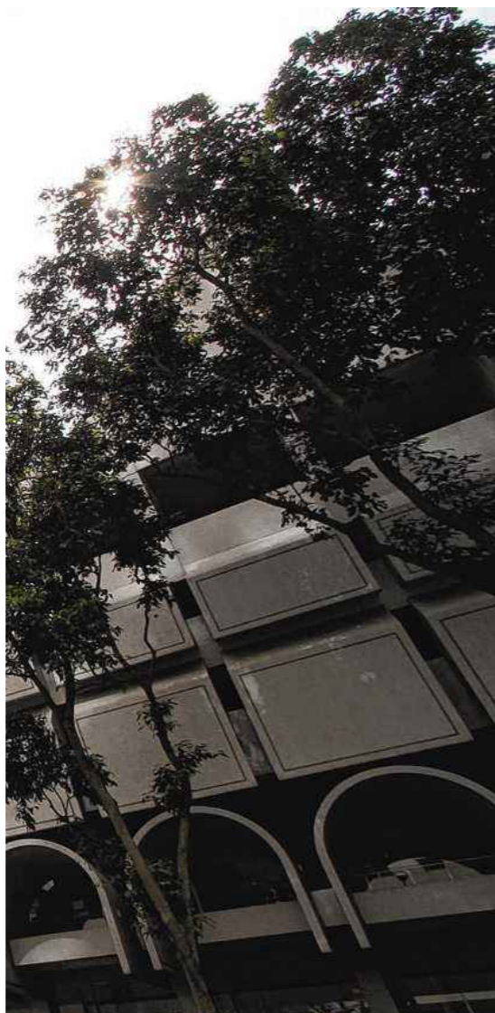
BEFORE: UIC Building in Shenton Way was demolished to make way for a new structure with 60 per cent more floor space. PHOTOS: SINGAPORE LAND GROUP
