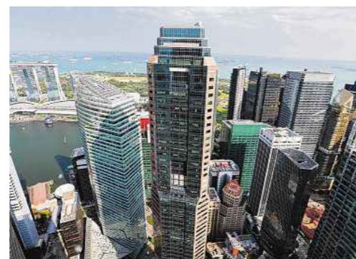
SPARED THE WRECKING BALL: Republic Plaza, currently tied for second-tallest building in Singapore, underwent a $70 million renovation in 2018. PHOTO: LIANHE ZAOBAO FILE
