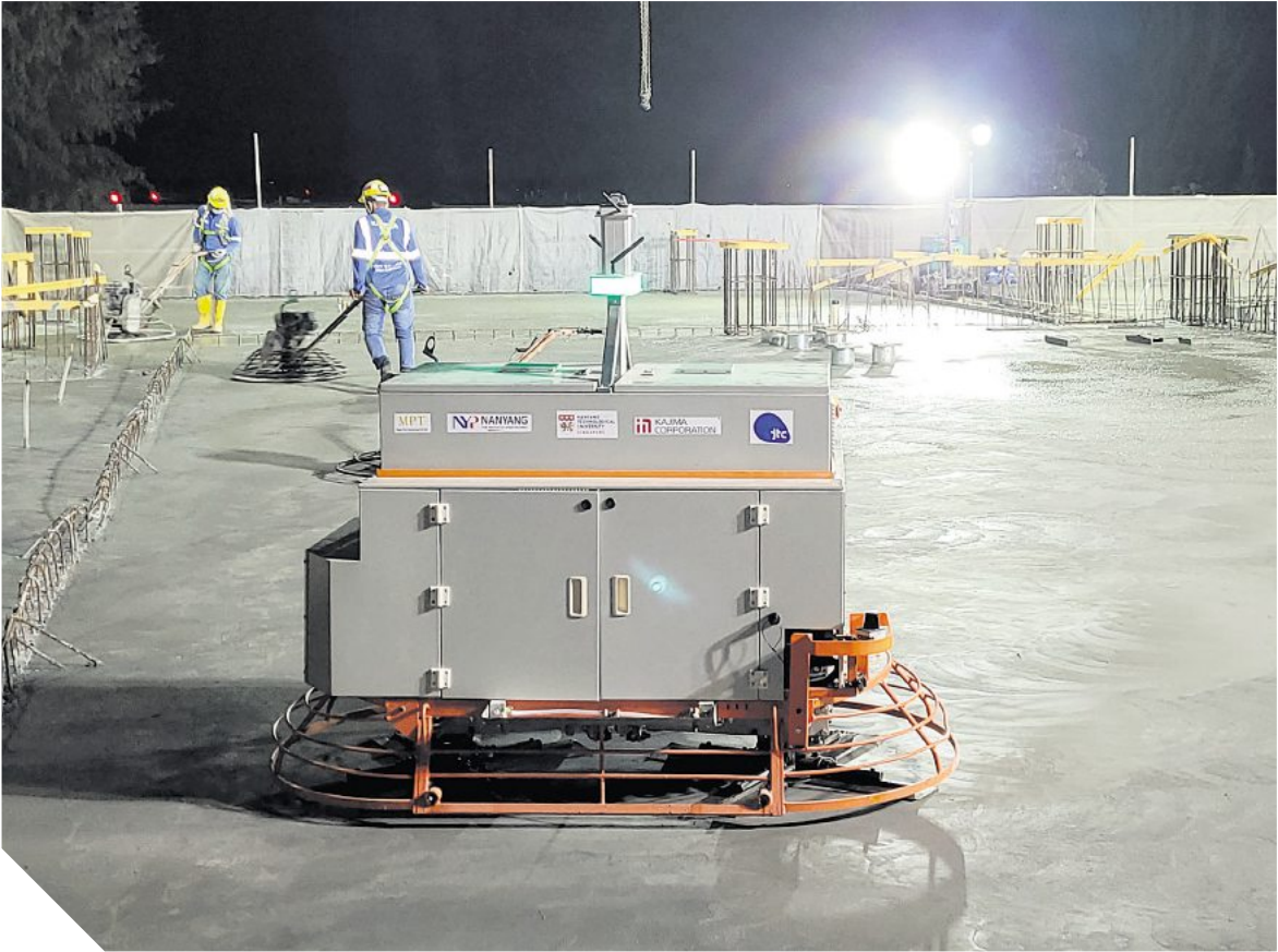
▲ Co-developed by the Kajima Technical Research Institute Singapore and its partners, the concrete finishing robot played a key role in building Kajima's Innovation hub, The Gear. PHOTO: KAJIMA CORPORATION
