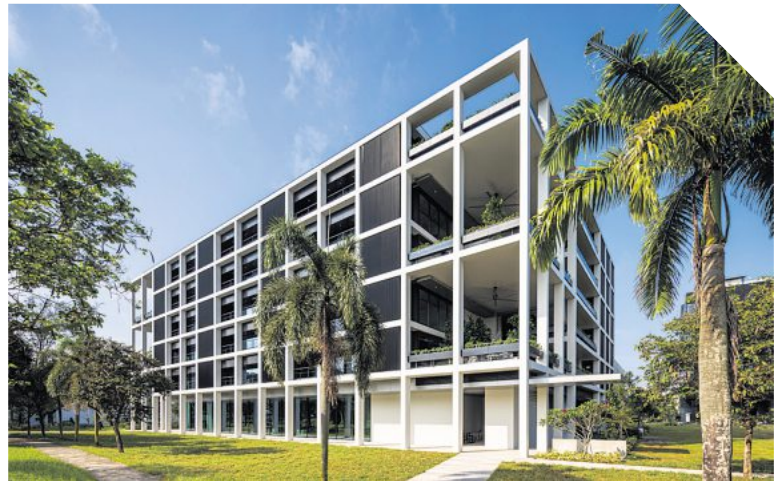
▲ The Gear, Kajima's six-storey hub at Changi Business Park, supports collaboration and growth among start-ups and corporations. PHOTO: KAJIMA DEVELOPMENT
